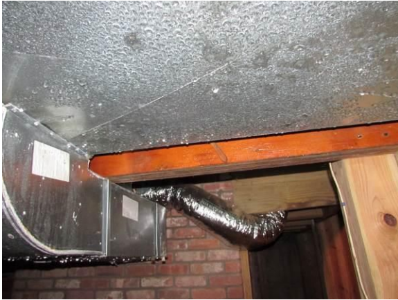
Photo No. 11: The basement is very wet from condensation, tidal flooding, and general humidity.
