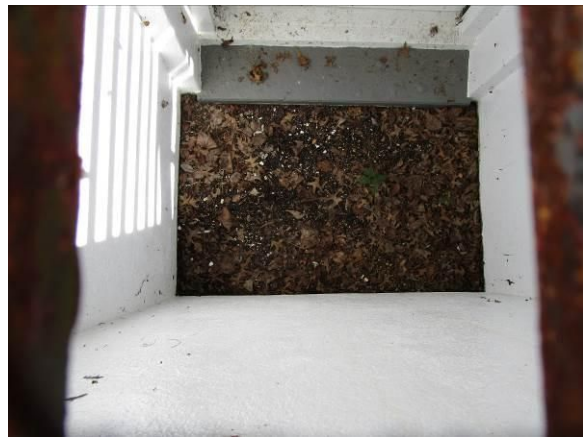
Photo No. 8: The window wells are a weak spot in water drainage management, despite recent improvements.
